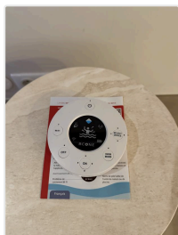
Control box, behind the living-room sofa.
